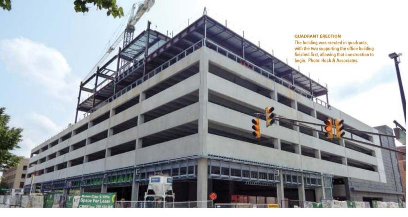
to open up visibility throughout the space while still meeting our loading requirements." Perimeter shear walls took most of the load, using splice sleeves to connect them. "It was easy to construct them but challenging to coordinate all of the loads for lateral resistance."
