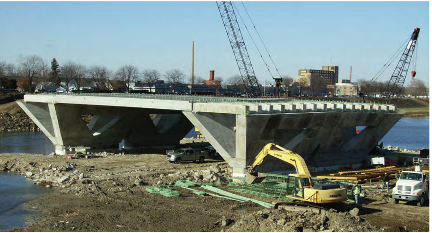
Solid, 42-in.-deep, precast concrete beams tie the legs of the Y-shaped piers and butt against the ends of 48-in.-deep, precast, prestressed concrete box beams spanning from pier to pier.
