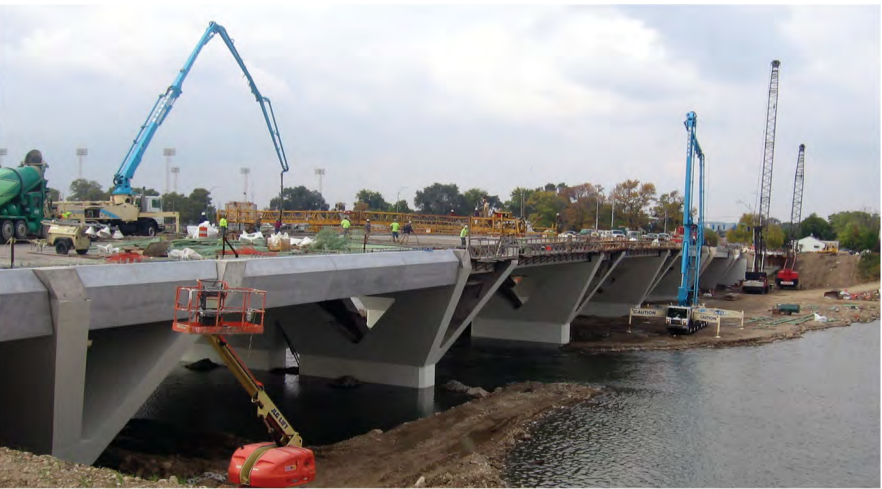
The dramatic effects of the precast concrete fascia panels can be seen during their installation.
