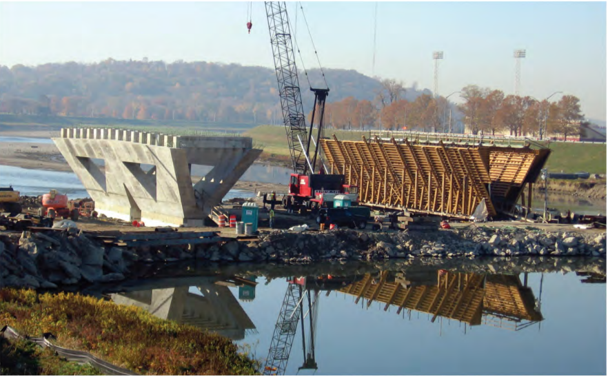
Legs of the Y-shaped piers are tied transversely with cast-in-place concrete box girders and longitudinally with precast concrete solid beams.
