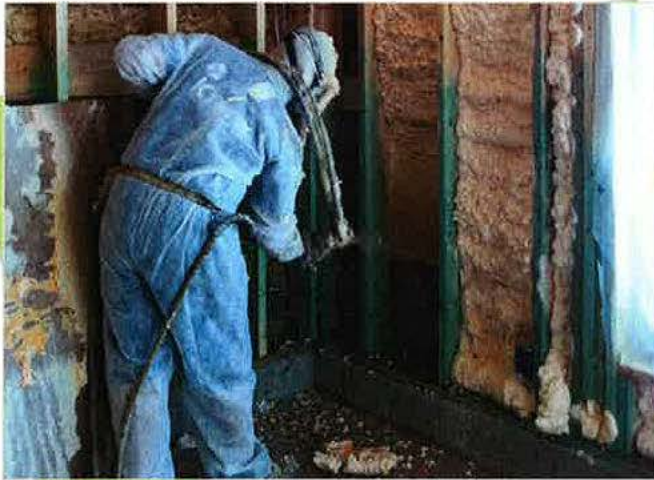
A worker sprays foam into the walls of the addition at AFCEE employee Erica Becvar's home to improve energy efficiency.
