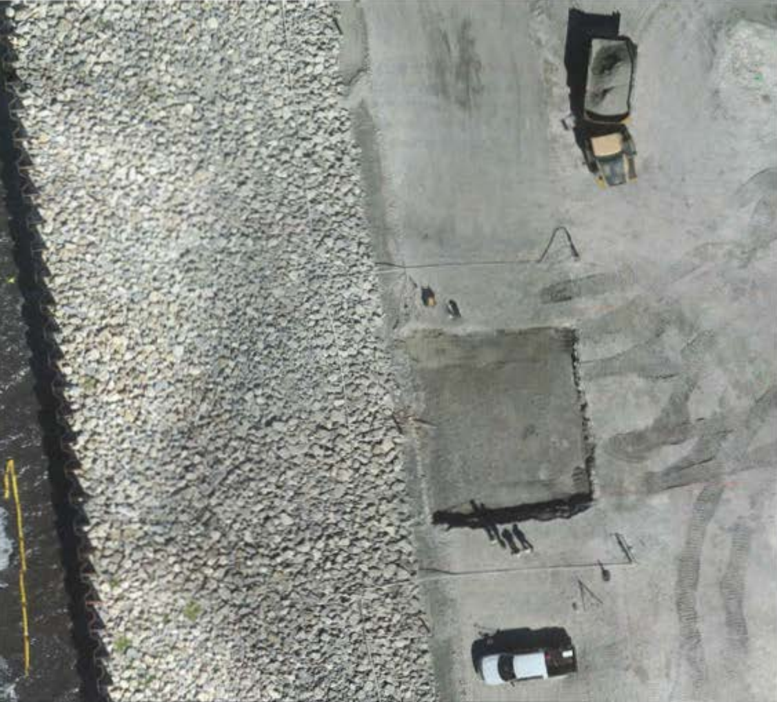
LEFT: UAS can help with construction management; at this levee in Florida, Woolpert's UAS collected high-resolution, accurate imagery at 1.5 centimeter resolution at an altitude of 128 meters AGL.
