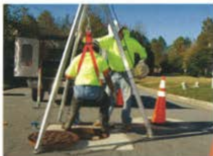
Woolpert staff installing permanent flow meter network.
