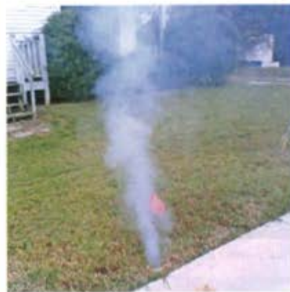
Smoke rises from a service lateral with a missing clean-out cap, located on private property in Gwinnett County. Smoke testing, performed by Woolpert, helped to locate inflow sources and defects in private laterals and connections. Gwinnett County used this information to develop a pilot program to educate private property owners about I/I and encourage them to voluntarily maintain their laterals and connections.
