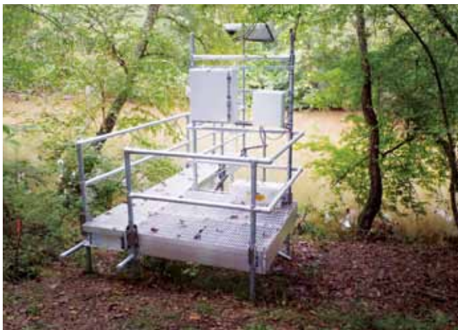
The flag-shaped design of the monitoring station creates a large work area, allowing multiple technicians to be on the platform together.
