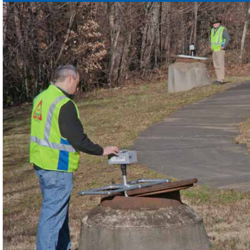
Utility crews using SL-RAT™ for inspections in the field.
