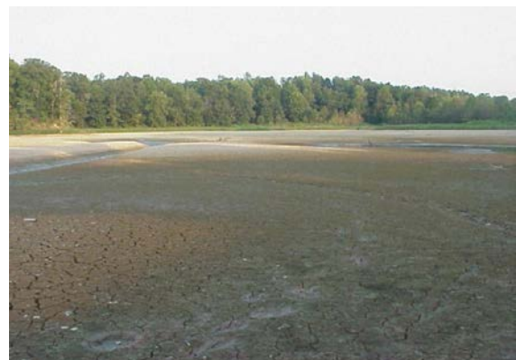
d. Substantial sedimentation behind Askalmore Watershed Dam, Tallahatchie County, MS.
