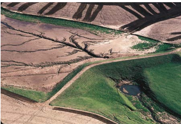
c. Grade-control dam on the Little Sioux River, near Sioux City, IA, caused significant sedimentation in the upstream water impoundment.
