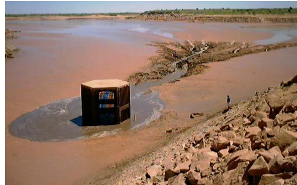
f. Reservoir sedimentation has buried the outlet at Sumner Dam near Fort Sumner, NM.
