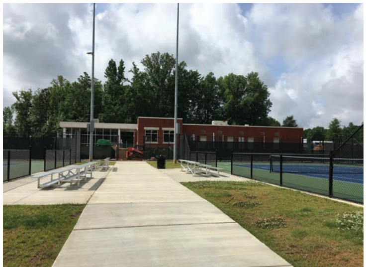
A VIEW OF THE REAR OF THE $1.7-MILLION, 6,200-SQUARE-FOOT QUEENS UNIVERSITY TENNIS CENTER AT MARION DIEHL PARK UNDER CONSTRUCTION.
