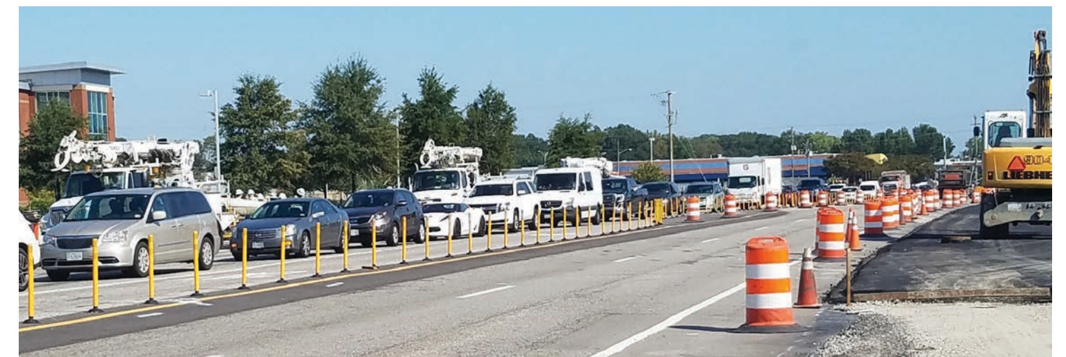
ABOVE: Woolpert conducted a traffic analysis for the MOT phases of the Witchduck Road project. Witchduck Road sees close to 60,000 vehicles per day.
