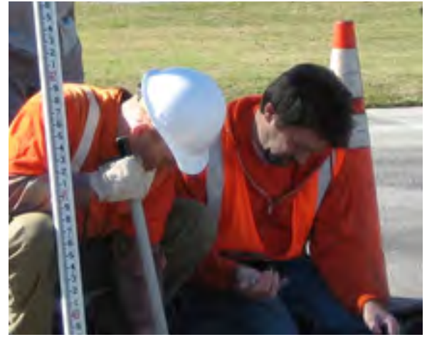
Figure 1: Inspecting sewer flow
